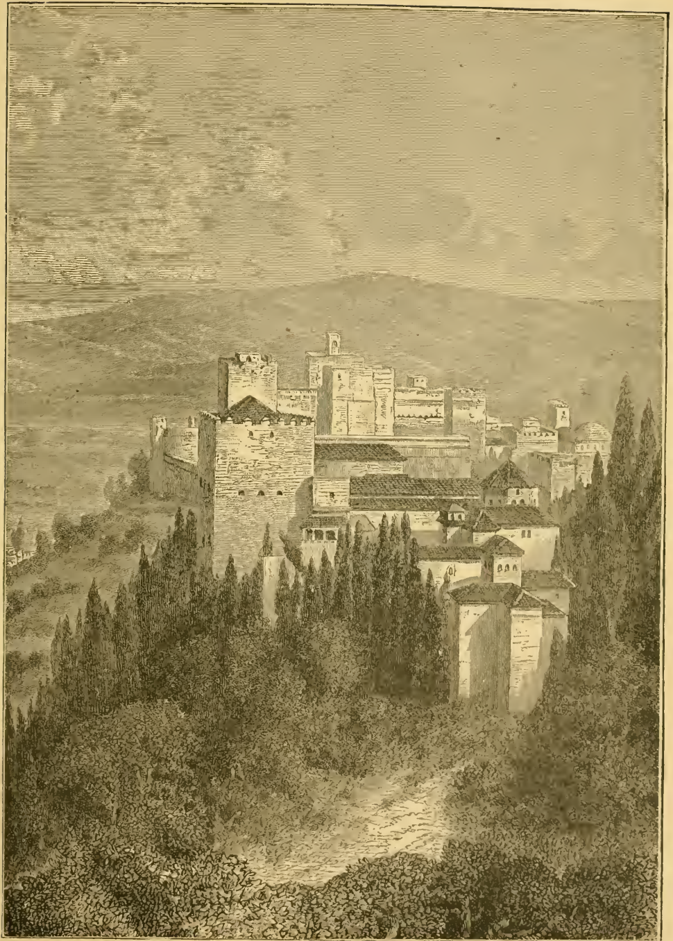
GENERAL VIEW OF THE ALHAMBRA.
